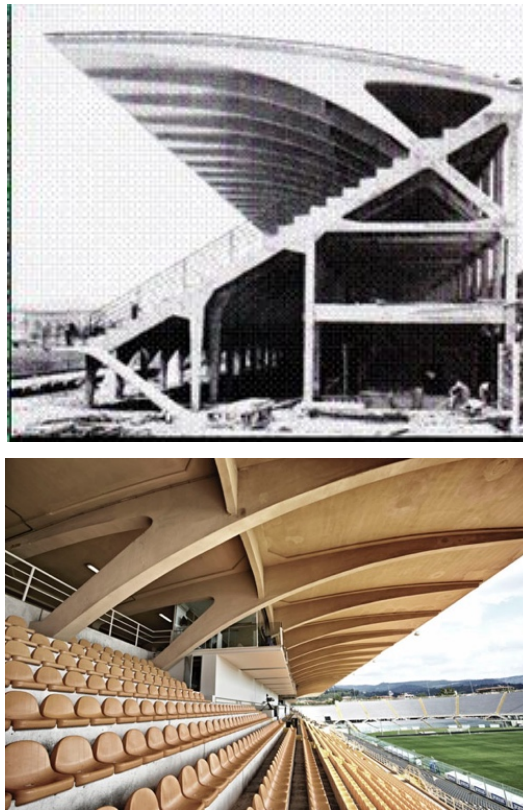
Figure 4.2: Top: side elevation of the integrated roof grand stand structure (book Ingg. Nervi & Bartoli, societa per azioni). Bottom: recent photograph of the seating roofed over by the cantilever.
